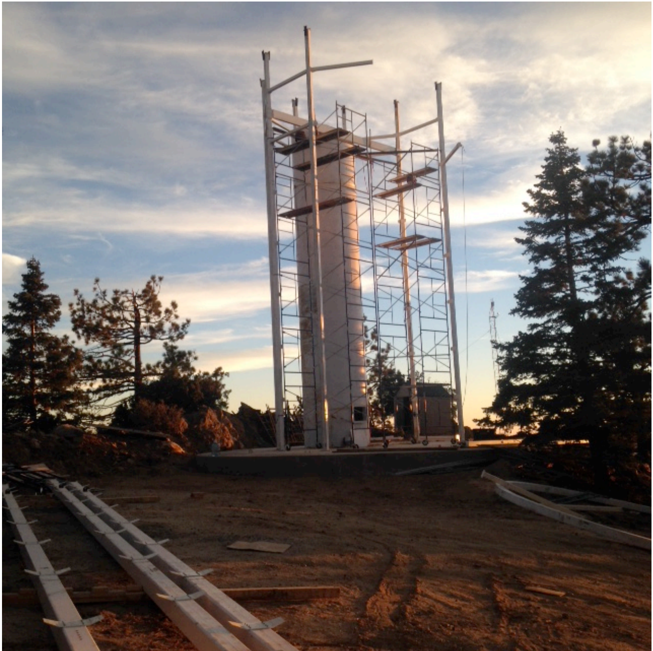
Site #1 Observatory Erection September 6, 2016
